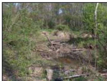
Stream Debris Dams
