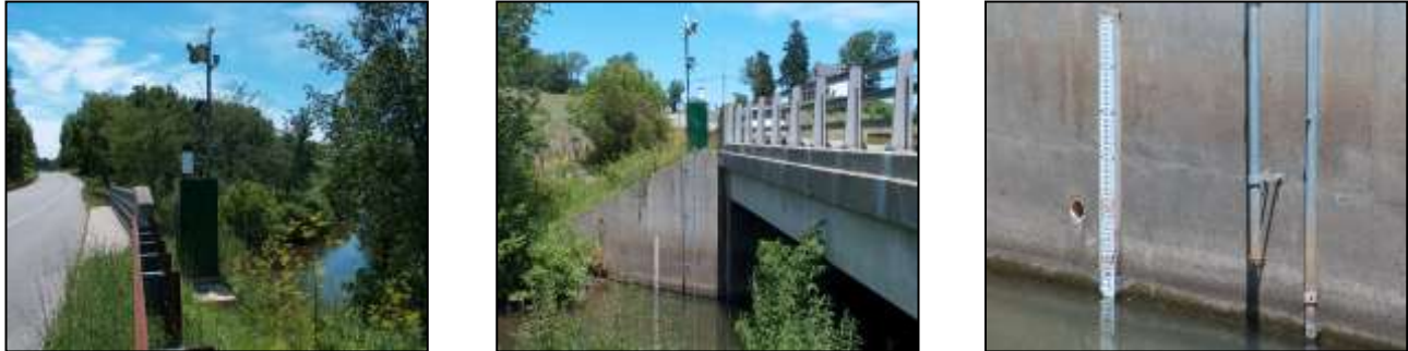
USGS Gage Station located on the Papakating Creek Pelletown Road, Frankford Township, NJ
